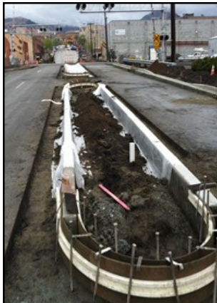
Orondo Street Improvement Project
